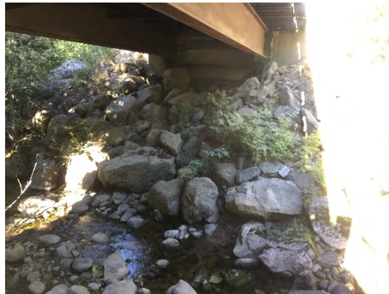
Right Bank Abutment when facing downstream
