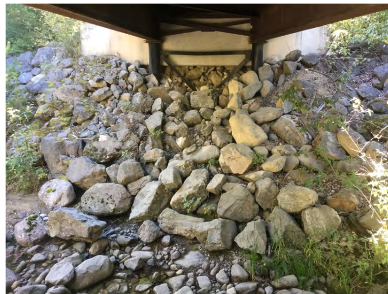
Left Bank Abutment when facing downstream
